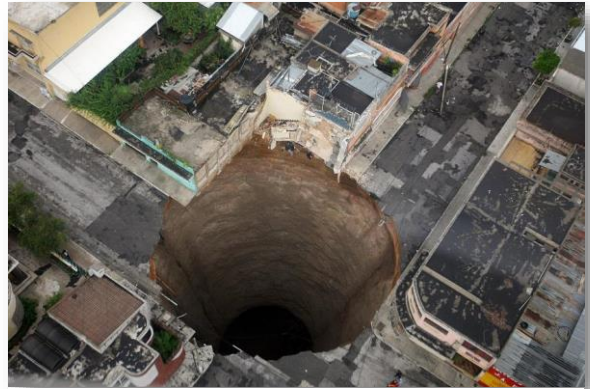
Sinkhole in Tampa, FL, circa 2013
